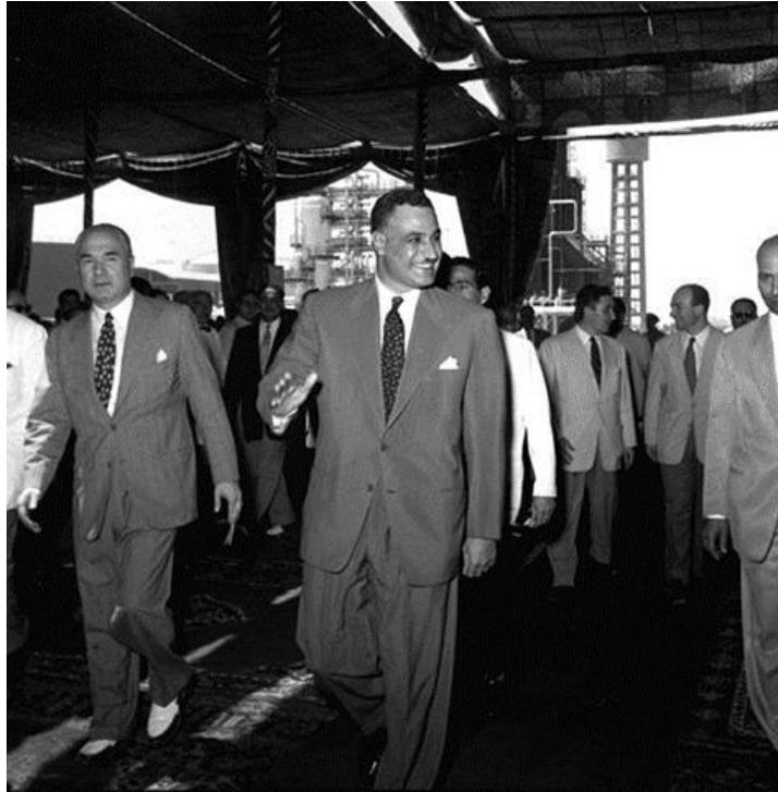
President Nasser inaugurates the oil pipeline in Musturud, July 24 th , 1956
